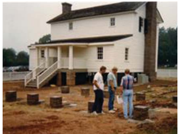
The piers for the detached kitchen house being inspected
