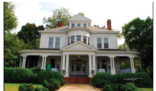
The Anderson House
